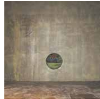
RC薬品貯蔵槽
